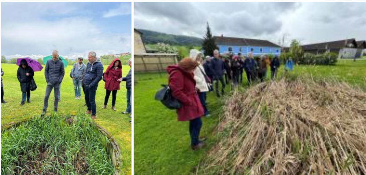
Figure 15: Planted sludge drying bed for SBR designed for 20 PE (plant 2, left) and Vertical Flow wetlands designed for 9 PE (plant 3, right).
