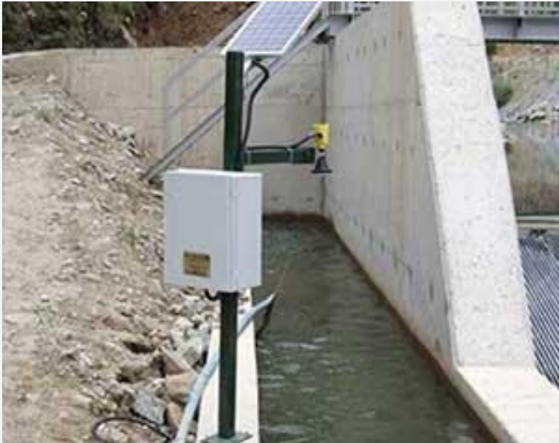
Stream Gaging Station
