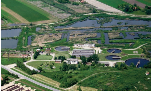
Water treatment plant from 2010
