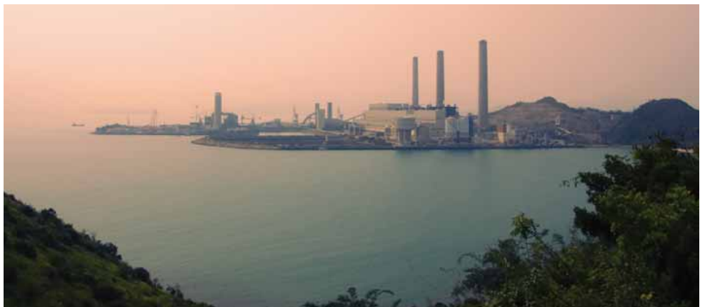
Lamma Power Station, Hong Kong, China. Thermal power stations use steam generated by heating water to turn the turbines that drive the generators. They also use copious quantities of water to cool the infrastructure, which is why so many are sited next to lakes, rivers or the coast. Source: Photo by Ben Tatlow on Unsplash.
