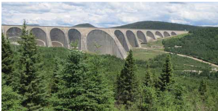
• Daniel-Johnson Dam, Manicouagan River, Quebec, Canada. The Daniel-Johnson Dam impounds the Manicouagan River and is the primary dam forming the Manicouagan Reservoir. It supports a major hydroelectric power station called Manic-5. Source: guyval [CC BY-SA ( https://creativecommons.org/licenses/by-sa/3.0/ )]
