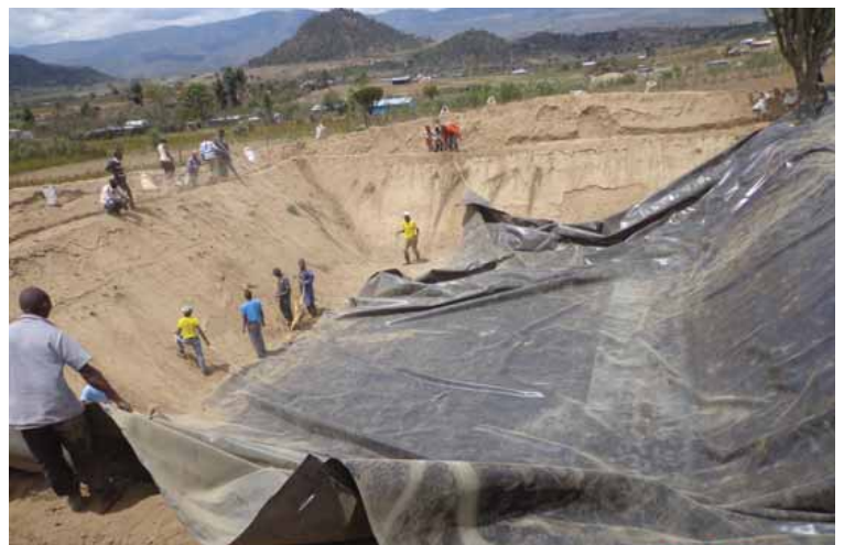
⚙️ Earthen barriers, or bunds. Whilst earthen bunds are common, some dam constructions are more substantial. Here we see the fixing of a liner over earthen barriers. Source: Syryjagu (CC BY-SA ( https://creativecommons.org/licenses/by-sa/4.0/ ))
