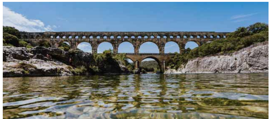
✦ Pont du Gard aqueduct, Gard, France. The Pont du Gard is an ancient Roman aqueduct bridge built in the first century AD to carry water over 50 km to the Roman colony of Nemausus. It crosses the Gardon River near the town of Vers-Pont-du-Gard in southern France. The Pont du Gard is the highest of all Roman aqueduct bridges, and one of the best preserved. Source: Xuan Nguyen on Unsplash.
