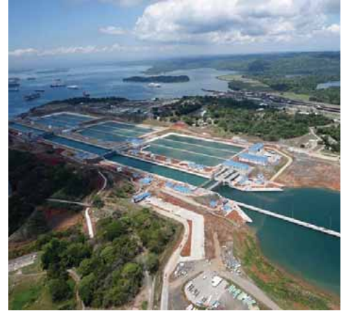
✦ Panama Canal, Panama. Agua Clara Locks, Gatun (viewed from the Atlantic side) before entering Gatun Lake, a large artificial lake (created between 1907 and 1913 by the building of the Gatun Dam across the Chagres River) that forms a major part of the Panama Canal. Source: US DOT (Public domain).
