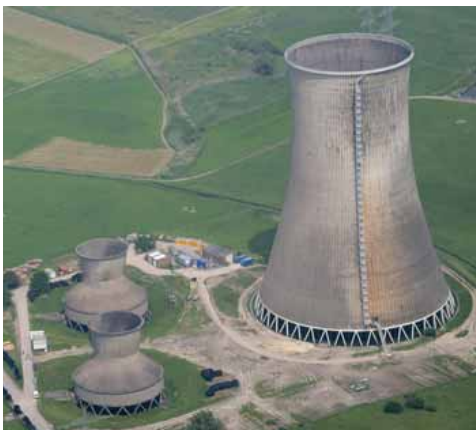
Power cooling towers, Westfalen, Germany. Forced draft wet cooling towers (height: 34 m) and a natural draft wet cooling tower (height: 122 m). Thermal electric power generation requires huge quantities of water to condense steam from the turbine exhaust. Source: Tim Reckmann [CC BY-SA ( https://creativecommons.org/licenses/by-sa/3.0/ )].
