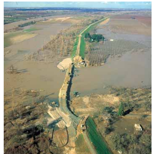
✦ Broken levee on the Feather River, California, USA. Aerial view of a broken levee under repair by U.S. Army Corps of Engineers on the Feather River near Nicolaus, California, USA. Source: Michael Nevins, U.S. Army Corps of Engineers (Public domain).
