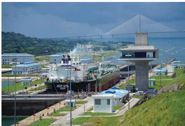
••• A ship passing through the Agua Clara locks. The dimensions of the Panama Canal's locks determine the maximum size to which many ships are built. These are referred to as Panamax and New Panamax vessels. Dimensions are fixed by the Panama Canal Authority, which issues regular notices to shipping (each January, or when otherwise required) 10 . Source: By Mariordo (Mario Roberto Durán Ortiz) - Own work, CC BY-SA 4.0, https://commons.wikimedia.org/w/index.php?curid=82643323
