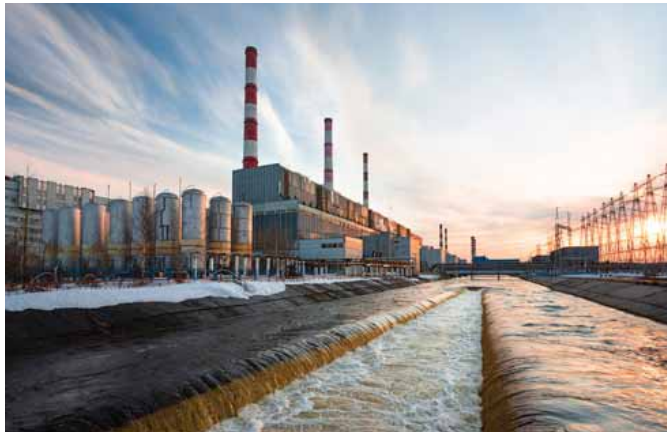
Surgut Power Station, Russia. Heated water cannot be returned directly to seas, lakes and rivers without harming the biosphere, so thermal power stations are sometimes accompanied by artificial lakes used for cooling before returning. Source: dedmaxopka@gmail.com
