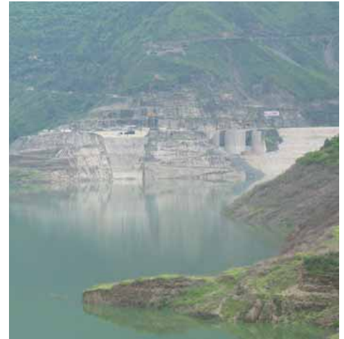
••• Tehri Dam, Bhagirathi River near Tehri Uttarakhand, India. The Tehri Dam on the Bhagirathi River is a 260m-high rock- and earthfill embankment dam. The reservoir of the dam drowned the District headquarters of Tehri, which have now been shifted to New Tehri. Furthermore, as the Bhagirathi River is considered part of the sacred Ganges, it has created resentment in some communities, who claim that the sanctity of the Ganges has been compromised for the generation of electricity. Source: Jeevanegi [CC BY-SA (https://creativecommons.org/licenses/by-sa/3.0)]
