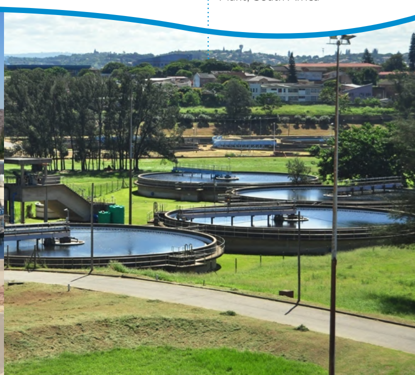
○ Durban Water Recycling Plant, South Africa
