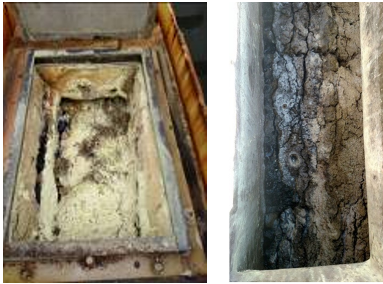
Figure 2.6 Thick and solidified scum layer inside different GLS separators of UASB reactors treating sewage (without proper removal devices and operational routines). Source: Chernicharo and Bressani-Ribeiro (2019) .
