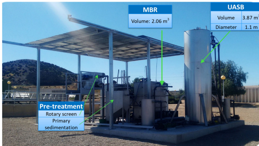
Figure 5.24 Image of the SIAM® prototype (using the second development) operated in the sewage treatment plant of the city of Cartagena (Spain), in the frame of the European Union Life Siamec project.
