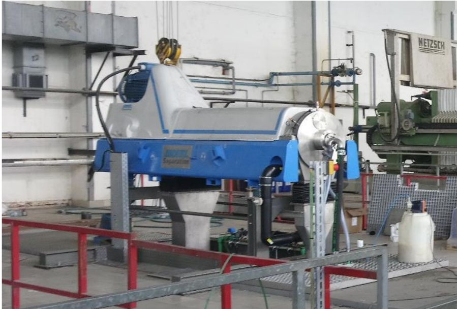
36. Figure: Dewatering in the North-Budapest WWTP
