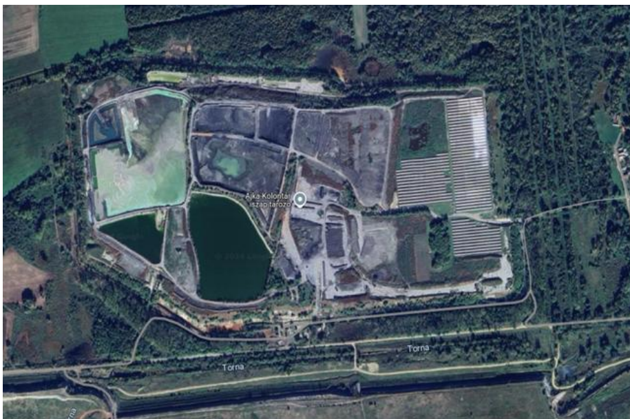
40. Figure: A former EWC-H plant near Ajka under rehabilitation
