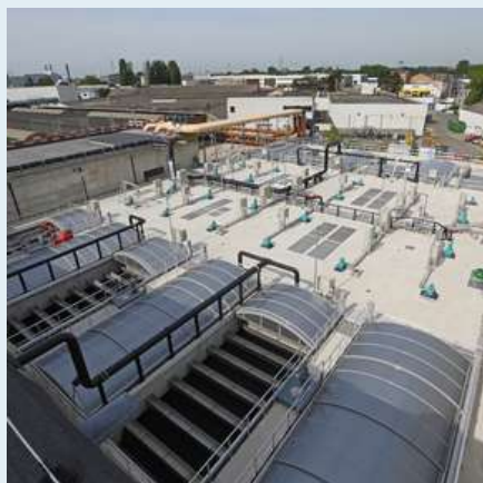
The recently renovated wastewater treatment plant 'Brussels South' managed by Hydria.
