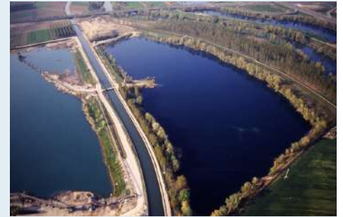
Lagoon basin near the Po river. Source: SMAT
