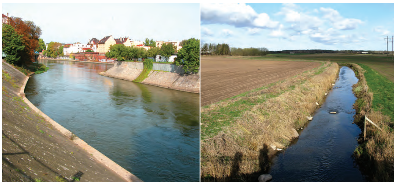
Image 3.2 Embankments for flood protection (left) and agricultural drainage (right)
