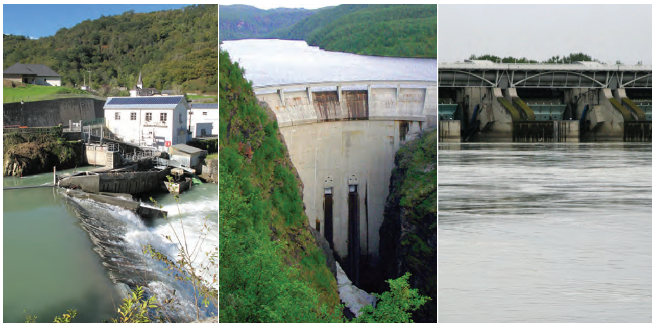
Image 3.3 Images of small hydropower plant (left) and large hydropower plants, storage, and run-of-river (centre and right)
