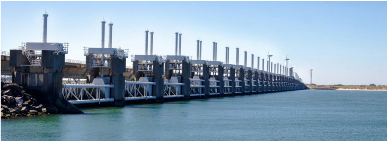
Figure 2: The Delta Works contribute to climate resilience by offering both short-term protection against extreme weather and long-term solutions for rising sea levels, ensuring that the Netherlands can thrive in a changing climate.
