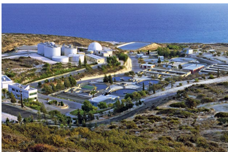
Figure CS3.1. View of the Limassol – Amathus water reuse system (Cyprus)
