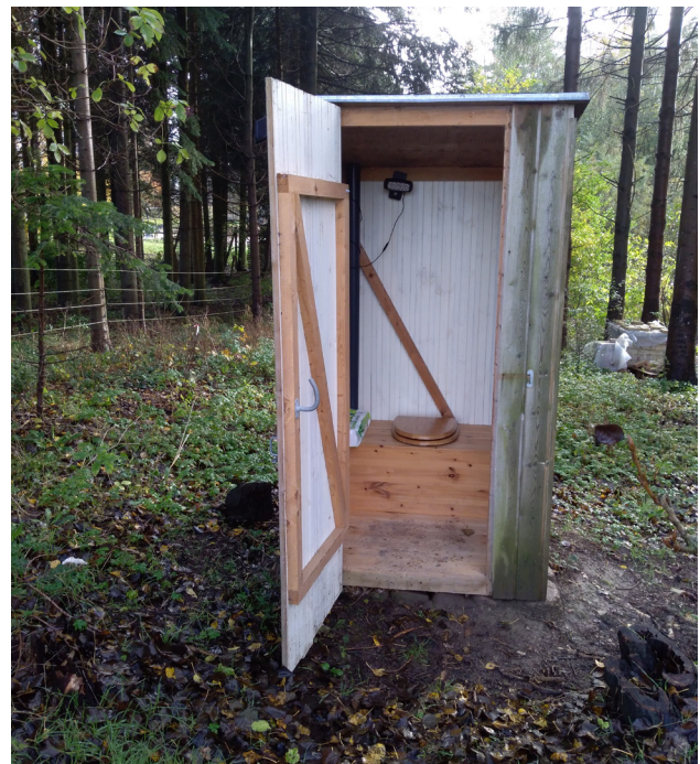
Image 2.2 A non-connected toilet, with a pit that requires emptying
