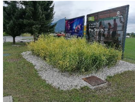
Petrol-pumping station (10 PE)
