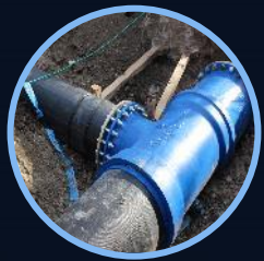
Incomplete metering of system's inlets and outlets
